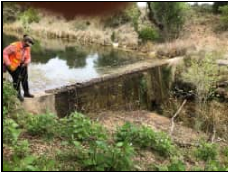
Figure 36. View of Resource 001 concrete dam, facing northeast
