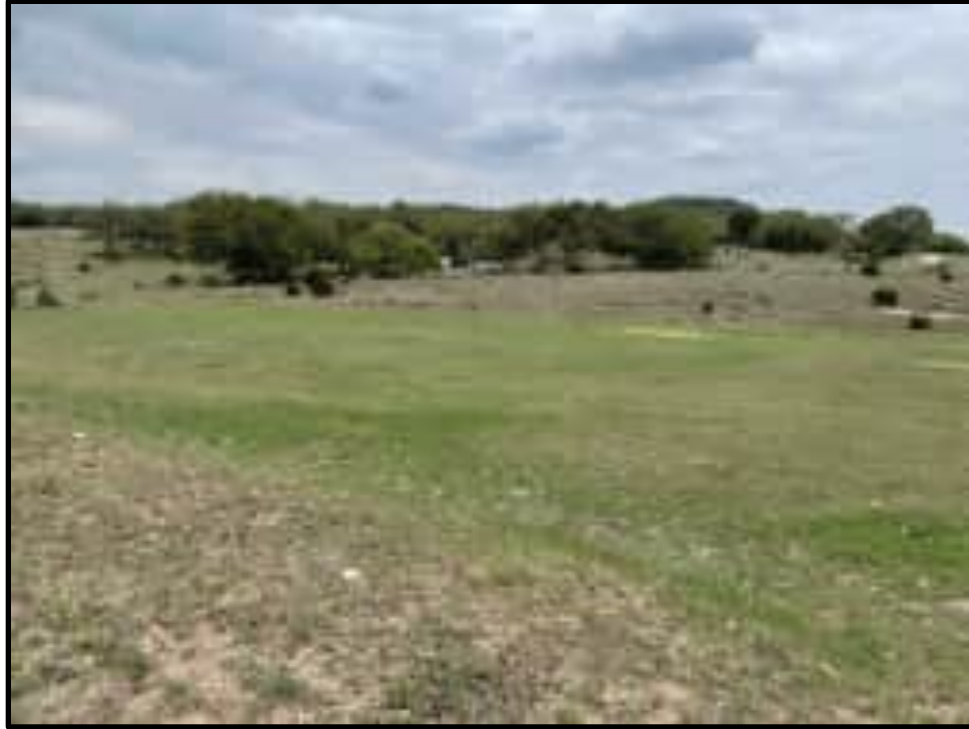
Figure 12. View of FRS No. 2 auxiliary spillway, facing north
