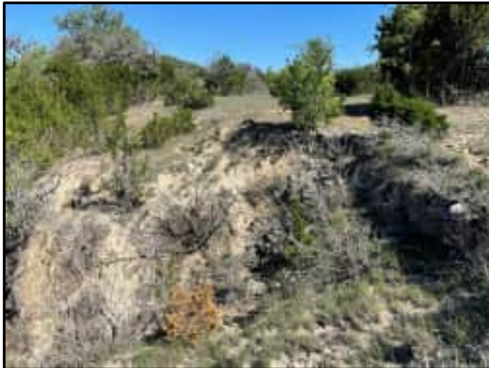
Figure 7. Erosion along high terrace scarp located north of Ranger Creek, facing southeast
