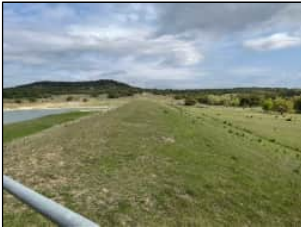
Figure 5. Overview of FRS No. 2 dam, facing north
