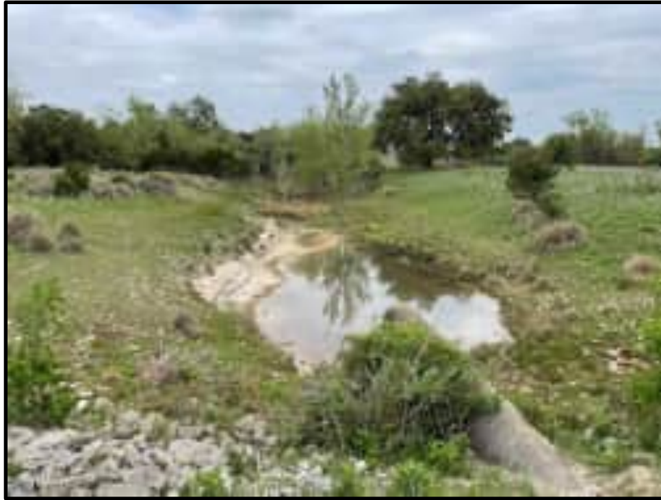
Figure 10. View of FRS No. 2 outlet pipe and plunge basin, facing east
