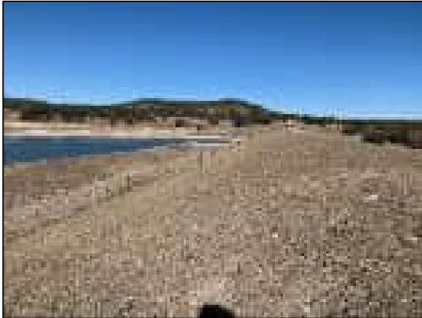
Upstream embankment and crown of dam (2020)
