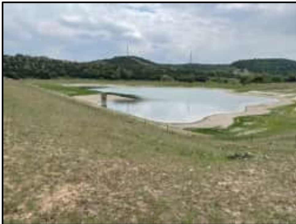
Figure 11. View of intake structure and impound area west of FRS No. dam, facing southwest
