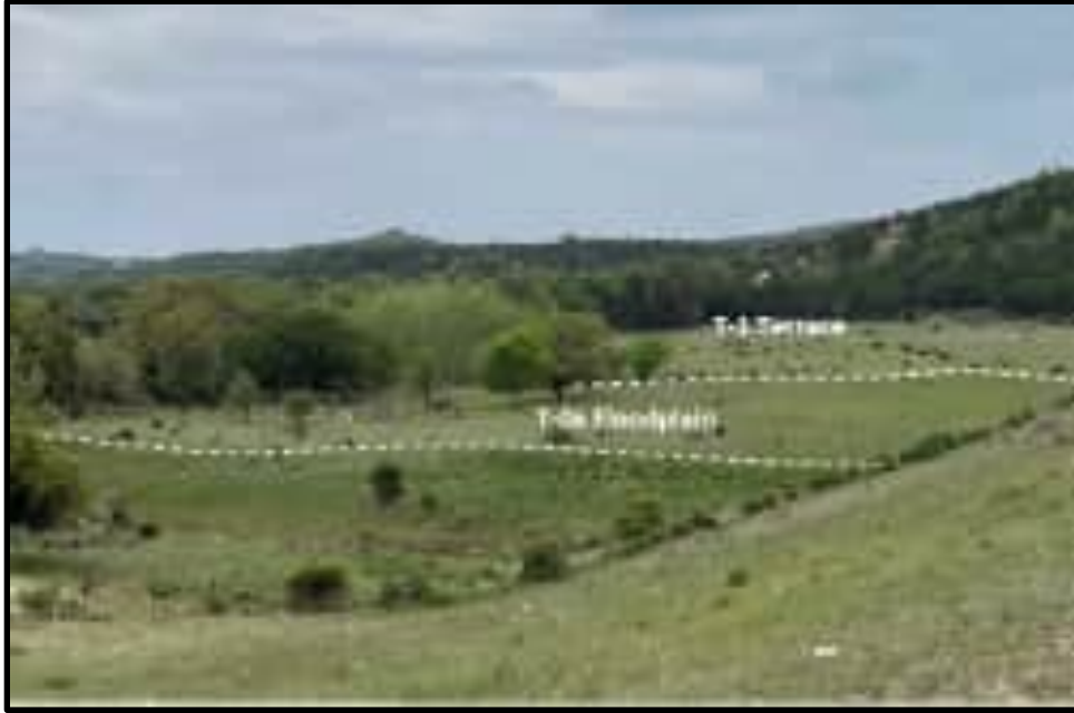
Figure 44. Overview of T-1 terrace, facing south from top of dam
